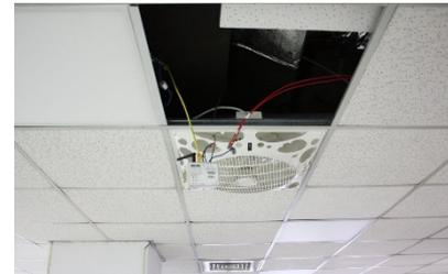
In the Fuli Township office, The light source was composed of 30W LED lights and 0-10V dimmable LED drivers. 4pc PIR sensors (SG100T) were installed near the office window, with the additional 89pc Indoor Lighting Control Boxes (SG200), 5pc Smart IoT Gateways (SG6200NXL), and 5pc Smart Energy Meter (SG3015) deployed across the office area to optimize energy efficiency.
