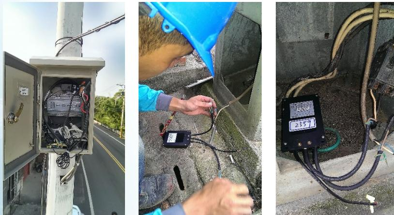
One SmartServer Segment Controller was installed a 2.4Km street section to control 50 geographically-scattered street lamps without any problem. SG7510 Intelligent Powerline Lighting Control Box was deployed underneath 50 street light fixtures to control power on and off, collect voltage and energy-saving data, and monitor street light status. No need for lifted trucks, drilling holes and can prevent unpredictable hot weathers.
