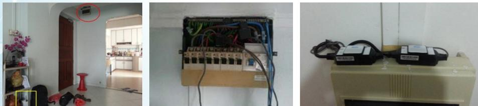
(2) One Smart Energy Meter SG3015-T3 and SG6200 Smart Energy Gateway were installed in per household.
