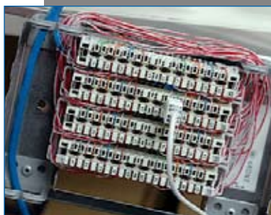
▲ This Krone block allowed us to change the length of the test copper phone line in 500m increments.
